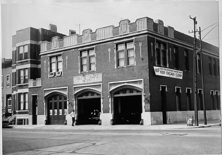
After PATROL 5 was disbanded in 1959, the city bought this building 1044 Orleans St for "special services" and is now quarters for the SNORKEL SQUAD NO. 1 which organized in late 1962.
