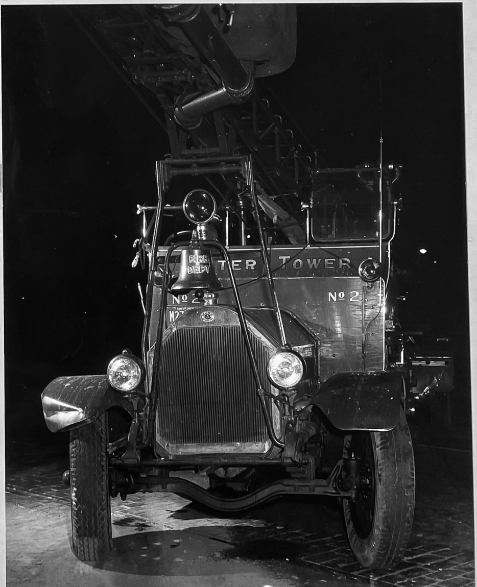
Water Tower - 2 May 4, 1960
