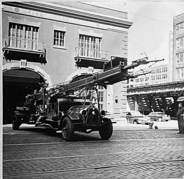
FORMERLY WATER TOWER No. 1 1928 SEAGRAVE 55 FT
