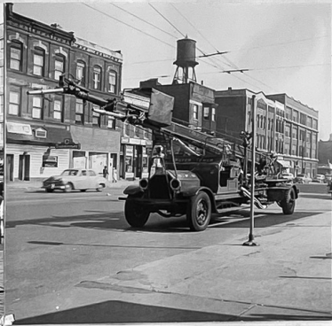
FORMERLY WATER TOWER No. 2 1925 SEAGRAVE 55 FT
