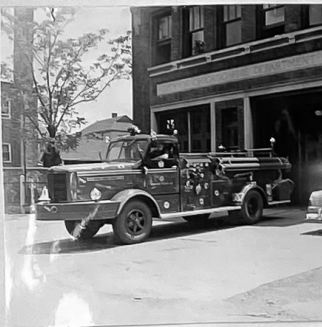
ENG 82 817 E. 91st St (BURNSIDE) 1953 FWD 1000 GPM
