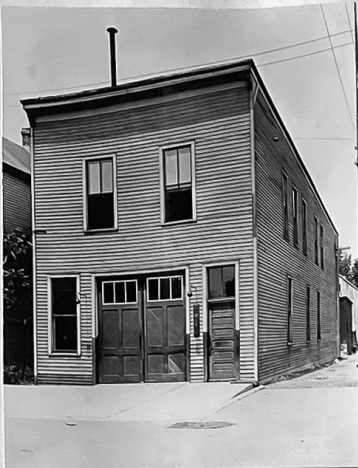
ENG 56 2214 Barry Avenue Occupied until June 14, 1936 and moved to TRK 21, 1529 Belmont Ave, and back to new house on same site on Dec 12, 1936.
