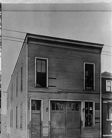
ENG 74 10615 Ewing Ave Organized and occupied until new building erected here on Aug 2, 1927.
